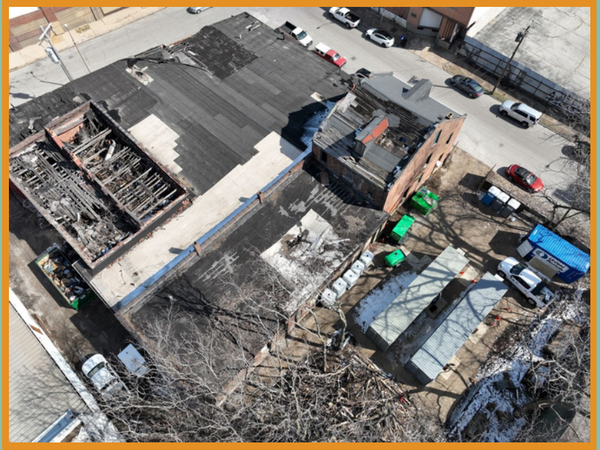
Aerial view of EPA cleanup at 2501 Texas
